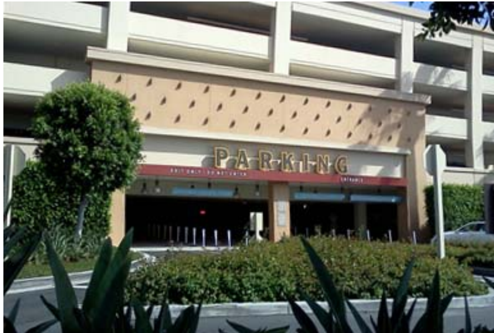
Figure 9-1 Parking Structure – DR testing
