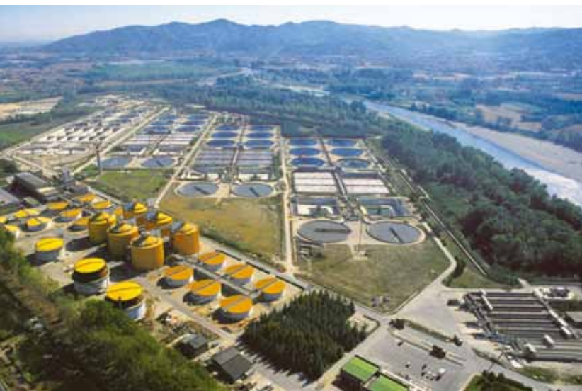
SMAT Castiglione, Turin: Greatest waste water treatment plant in Italy.
